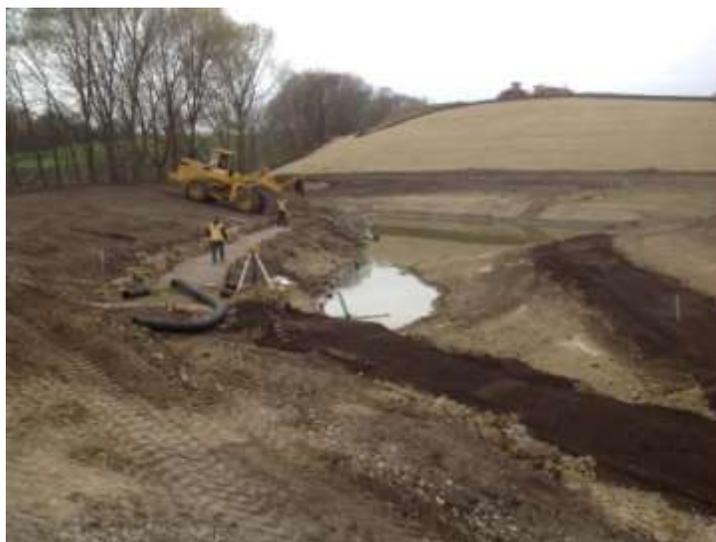
Installation of a bio-filtration bench on a new storm-water pond
